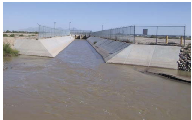
Figure 4. American Canal Extension
