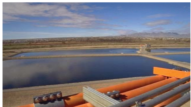
Figure 5. Presettling: 45 acres of presettling ponds provide 146 million gallons of raw water storage and remove 75% of the raw water turbidity.
